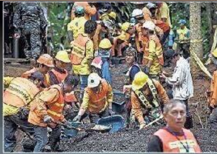
Workers fix the road leading to Tham Luang cave
